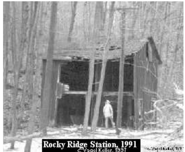
The author took this picture of the Rocky Ridge station, missing its southwest wall, in late-Autumn 1991 shortly before it collapsed.
