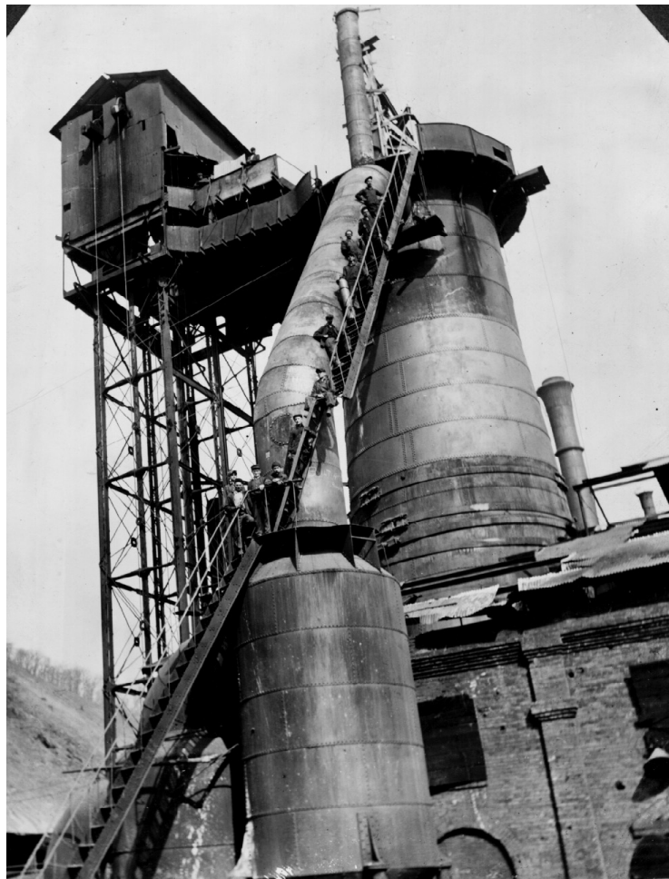
This view of one of the two coke-fired stacks of the Saxton Furnace, located on the west side of the Broad Top Coalfield, ca. 1910, shows the downcomer and dust catcher, as well as an elevator for lifting the charge to the top of the stack. The hot ovens are off scene to the left in this view. Photo courtesy of Jon Baughman.
