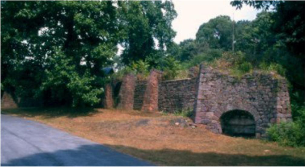
Iron ore for the Cornwall Furnace came from a nearby open pit mine. Before it was charged into the furnace, the ore was heated in these “roasters” to remove impurities. Cornwall iron ore was of a very high quality, and it was used in Bethlehem Steel’s blast furnaces at Bethlehem, Pennsylvania into the late 20th Century.
