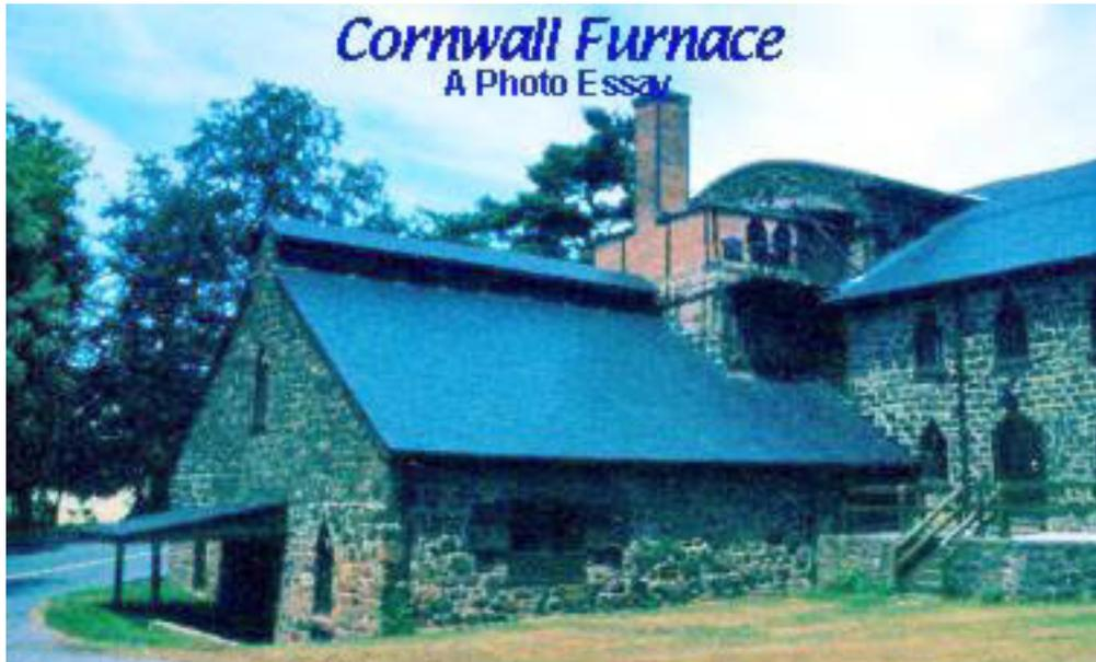
Cornwall Furnace is located in Lebanon County, east of Hershey and south of Lebanon, Pennsylvania. In the title view the stone cast house extends from the base of the blast furnace stack, which is almost completely hidden by the surrounding structures.
