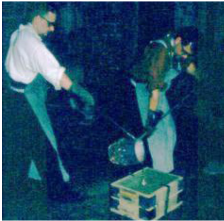
Besides wrought iron, iron plantations produced commercial castings for local markets. Here, a skilled molder employed by the Park Service and his park ranger apprentice perform a living history demonstration at the furnace. Wearing clothing appropriate for the early 19th Century (except for safety goggles and gloves) they take visitors through the process of making a mold and casting a part for an iron stove.
