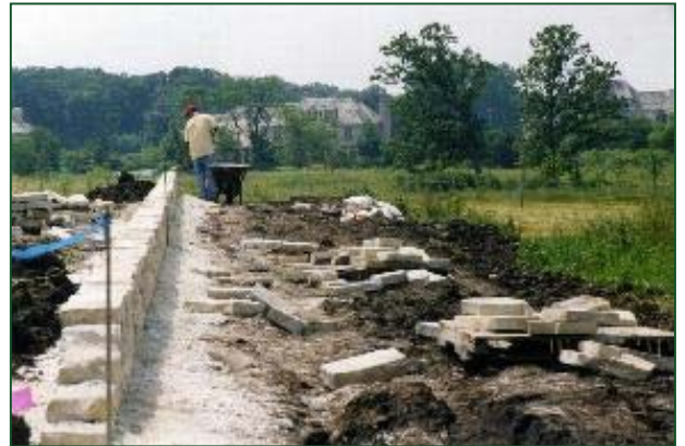
Stone ledges rebuilt, 2006
