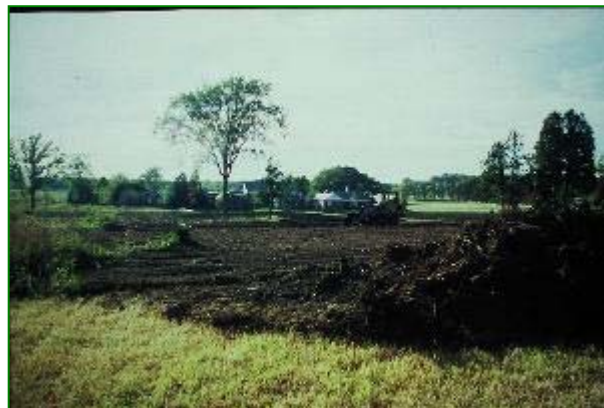
Campanella's bulldozer removing stumps and grading, 2004
