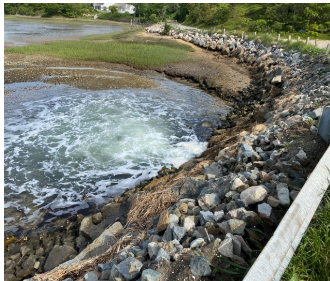
Figure 2 — Downstream Culvert Outlet and Stone Armor Slope Protection (Facing North)
