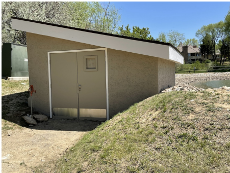
Refurbished pump house
