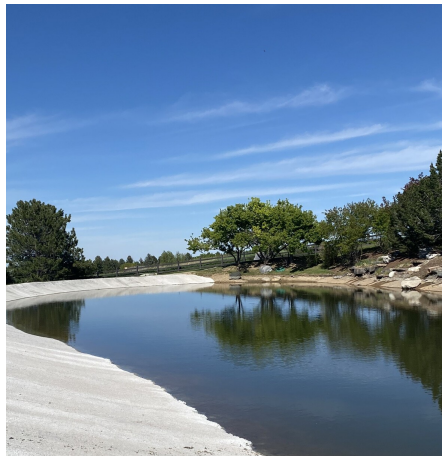
PARTIALLY FILLED POND
