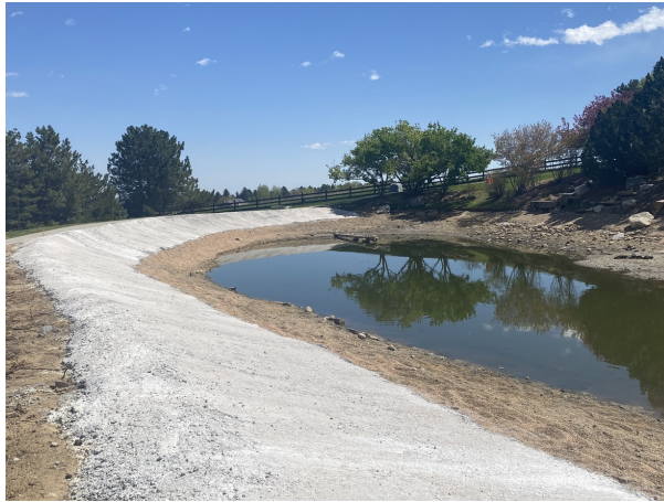
COMPLETED REPAIRS BEFORE FILLING
