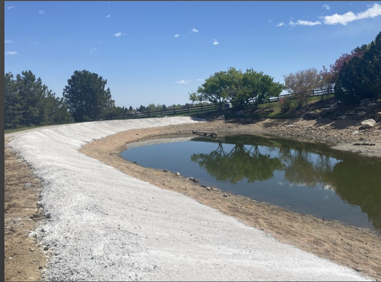
North side repair, concrete apron
