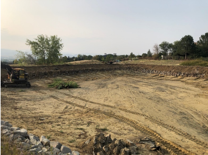
Sludge and old PVC liner removed, starting condition
