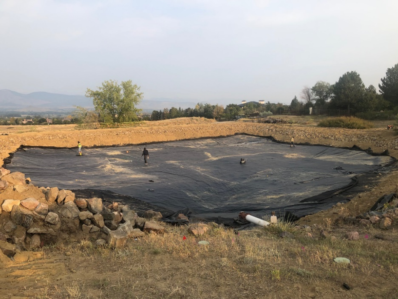
Liner in place, rip-rap sides unfinished
