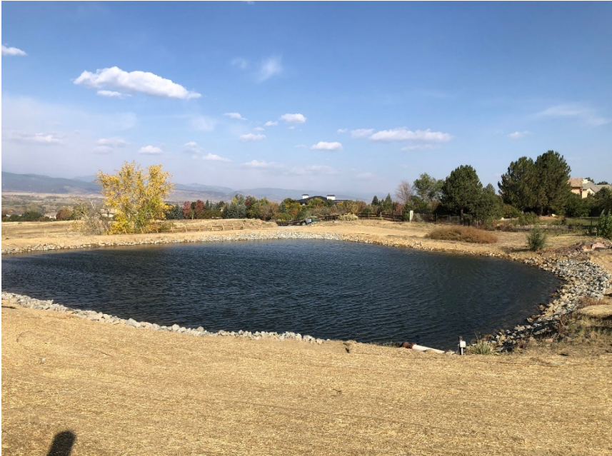
Pond completed and full, vegetation seeding blankets surround
