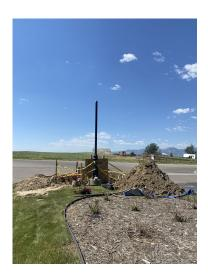
Upon starting the irrigation system, a large water leak was observed near the island at the entrance to the neighborhood off Highway 52 onto Somerset Drive. The mainline is greater than 6' below the road, so repair of this line required removal of the flowers (stored for replanting) and the light pole. The line has been repaired, but the grass on the east side of Somerset Dr from the entrance to the pool wasn't watered during the repair, which has led to extensive brown areas.
