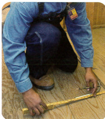
5. Mark conduit at the required stub-up length.
