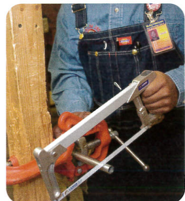
6. Cut conduit to length.
