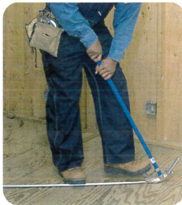
4. Use heavy foot pressure to make bend.
