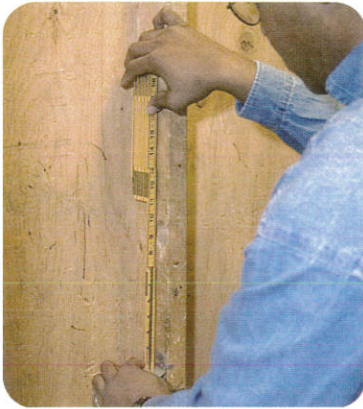
1. Measure stub-up length.
