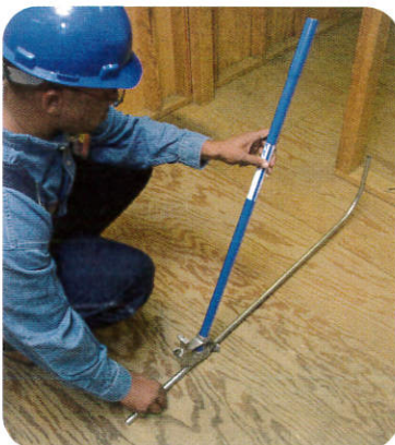
4. Make second bend at pencil mark and in same plane.
