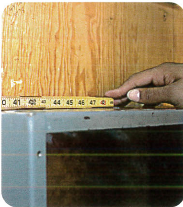
1. Measure between knockouts for the back-to-back distance.
