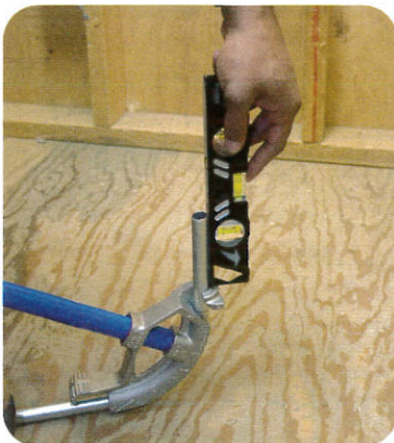
5. Check bend with torpedo level.
