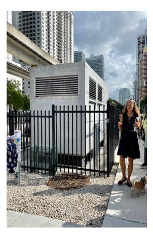
Picture of one of many stormwater pump stations fighting flooding conditions and rising sea levels on the streets of Miami and Miami Beach. Before stormwater pumps were installed, the water was carried out into the bay by the force of gravity. Due to sea level rise the water no longer flows by gravity to the bay. Instead the water flows back into the streets resulting in flooding. The existing pump stations redirect the water to the outfalls.
