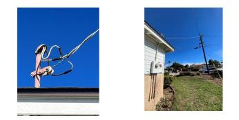
photo of the overhead riser, point of attachment, and service drop
