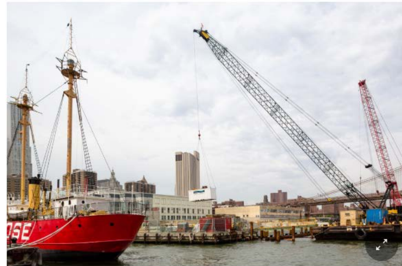
Construction at Pier 17 at the South Street Seaport. The Howard Hughes Corporation is spending $425 million to rebuild Pier 17 and erect a glassy four-story mall. Pablo Enriquez for The New York Times
