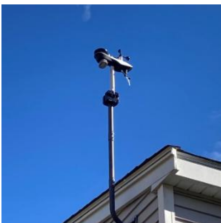
Installing the new weather station on the roof
