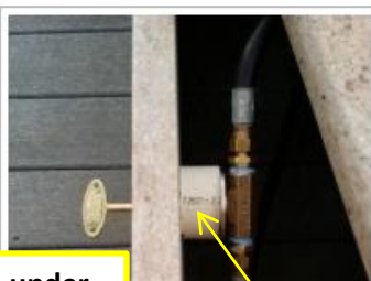
Use 1.5" PVC to shim back Key Valve.
