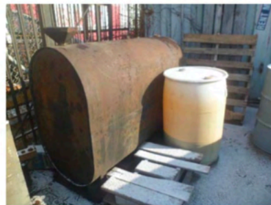
#12: View of a used oil AST located on the north side of the southwestern parking lot. Makeshift secondary containment was observed beneath the AST.
