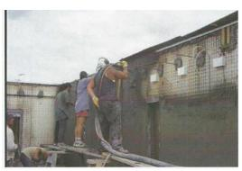
concrete for approximately 30 minutes and then start cutting and screeding as per required thickness. It is very important that concrete fill the whole area between the polystyrene and the reinforcing mesh (this is the most critical area to achieve a required strength). It is also important to fill all other gaps and voids during the application.
