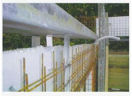
The correct height of the wall and their straight position must be accurately measured using and accurate laser instrument. Any adjustment must be done before concrete is applied to this area.
