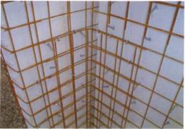
Additional reinforcing is typically added inside and tied to the mesh. Reinforcing used to increase the strength of panels (typically in floors) should be high strength steel - HD.
