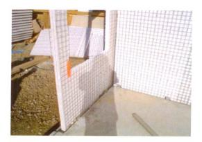
These bars may either be cast into the footings or drilled and epoxied in as the walls are erected, depending on accuracy of set-out. The starter re-bars are placed inside of the panels between the reinforcing mesh and polystyrene connected with tie wires to the mesh. Depending on the structural engineering design, in some locations, re-bars will be required to be installed on both sides of the panels.
