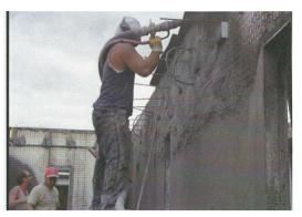
It is a good idea to start a shotcrete application on parallel walls first and then, removing the screed lines at the corner start with other parallel walls in the other way. With this scenario, it is likely to achieve a
