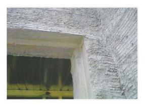
Metal frames are fixed to the panels using metal bracing which are placed in the line with openings and base U brackets. They are fixed using tech crews (metal to metal) fixings. Special attention must be taken for plumbing and straightening of the frames before concrete starts.
