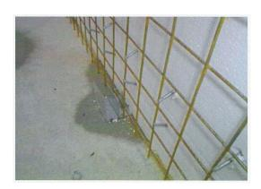
Once the U brackets are in place, the Smart Panels Walling System panels are installed inside of base U bracket, on top of the floor slab or foundation. The foundation and slab details are like that required when constructing a block wall or pre-cast panels. Starter rebars of 12mm diameter, spaced at 600mm centre must be installed for at least one side of the wall to attach the walls to the foundation or to the floor.
