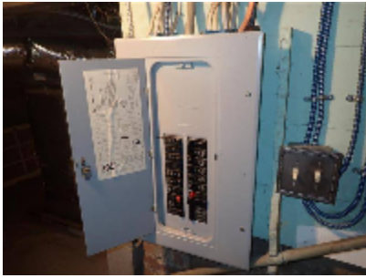
Electrical distribution panel in basement Main shut-off is located outside at the meter base Kitchen
