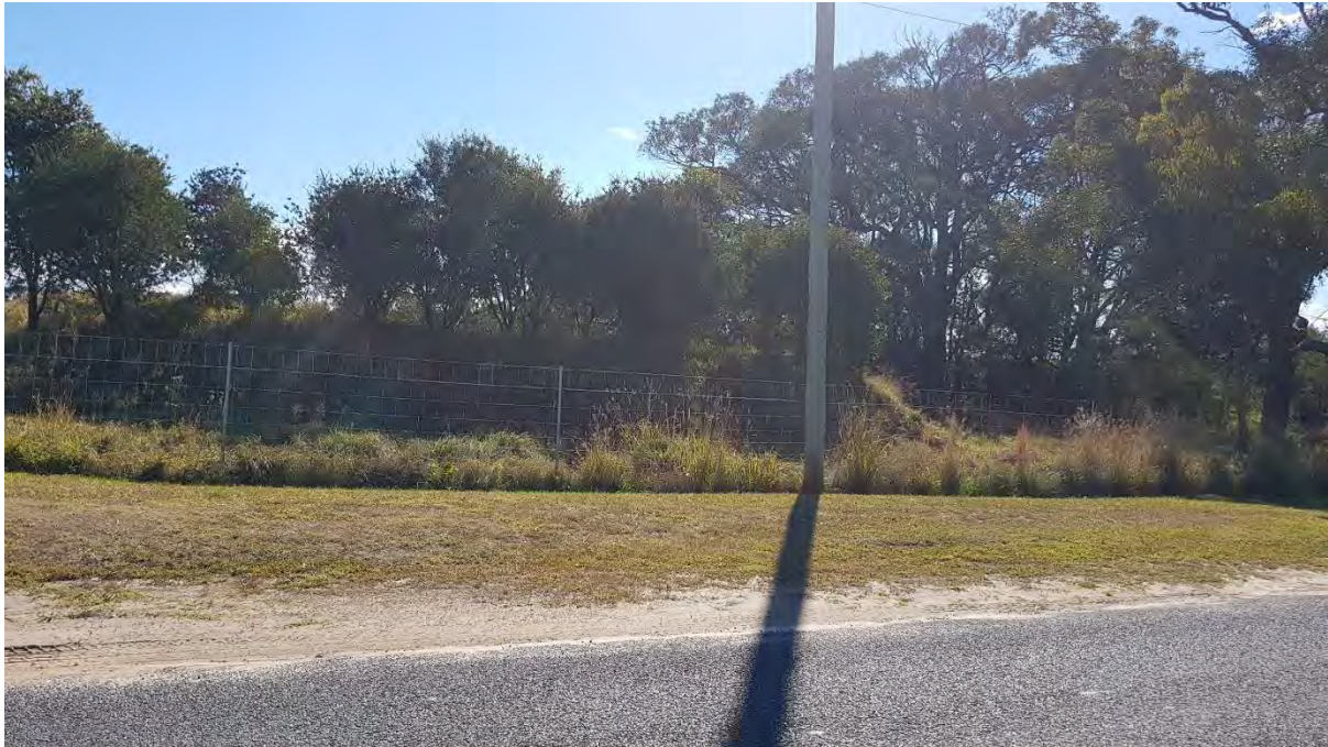
Figure 6. Bund wall immediately north of Roberts Road site entrance
