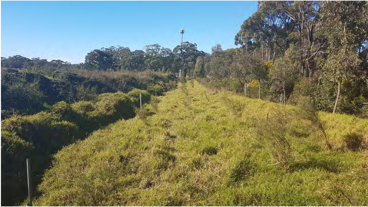
Figure 7. Planted native vegetation along Old Northern Road
