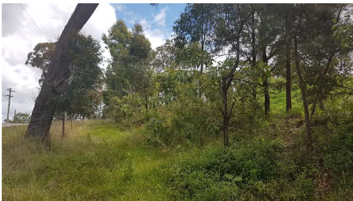
Figure 3. Bund wall adjacent to Roberts Road.
