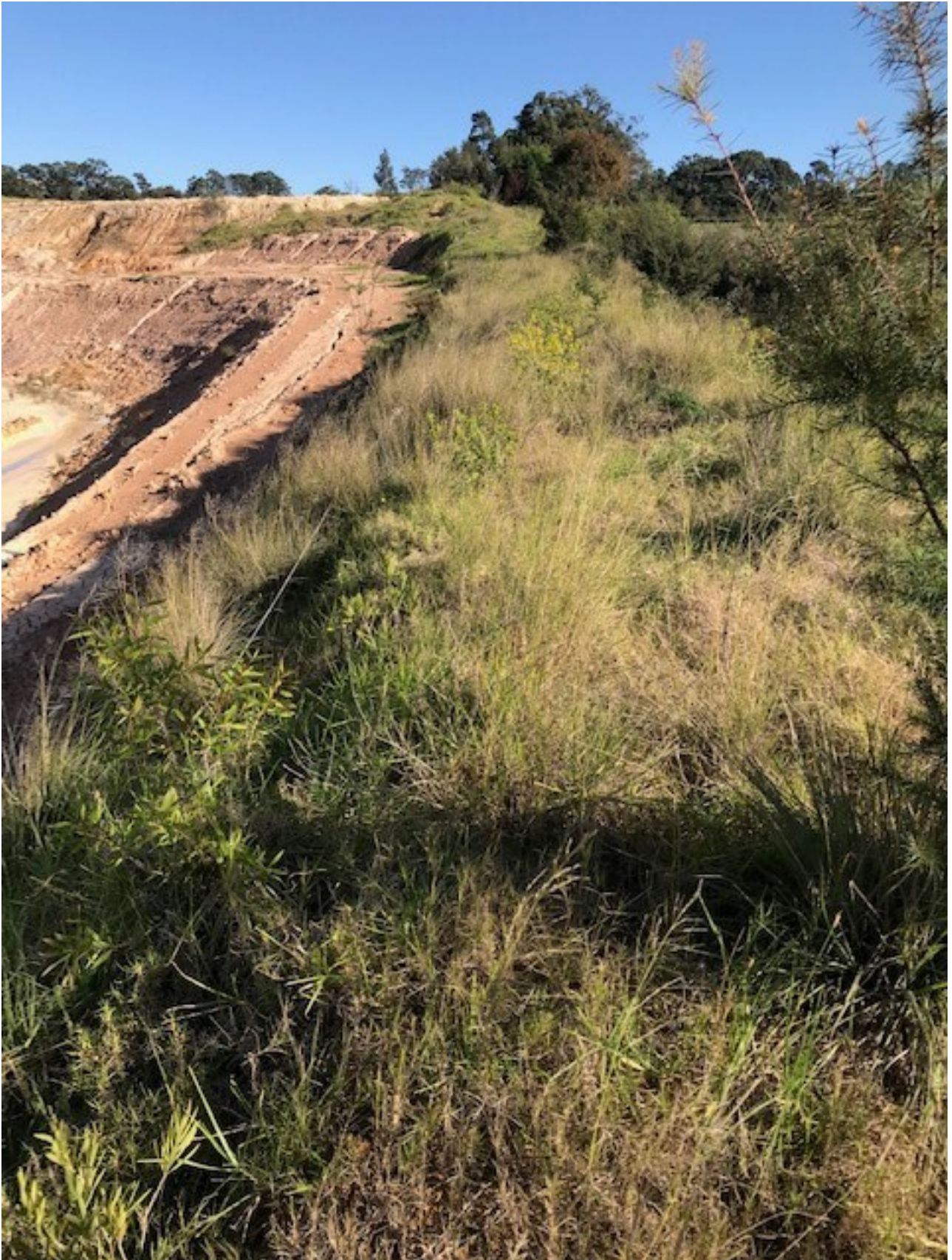
Plate 15 – Northern bund rehabilitation
