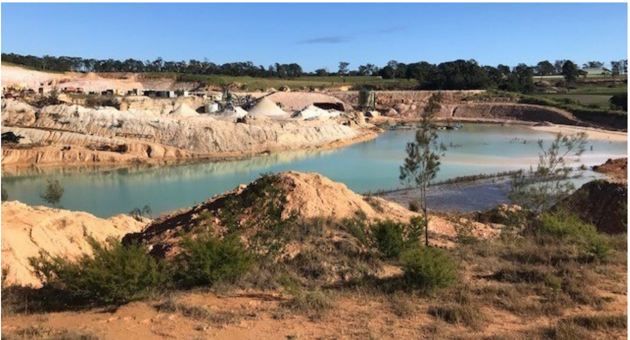
Plate 8 – Dam 1 process water
