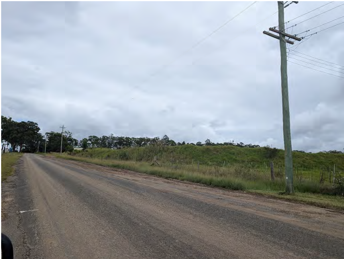
Figure 3. Bund wall adjacent to Roberts Road.
