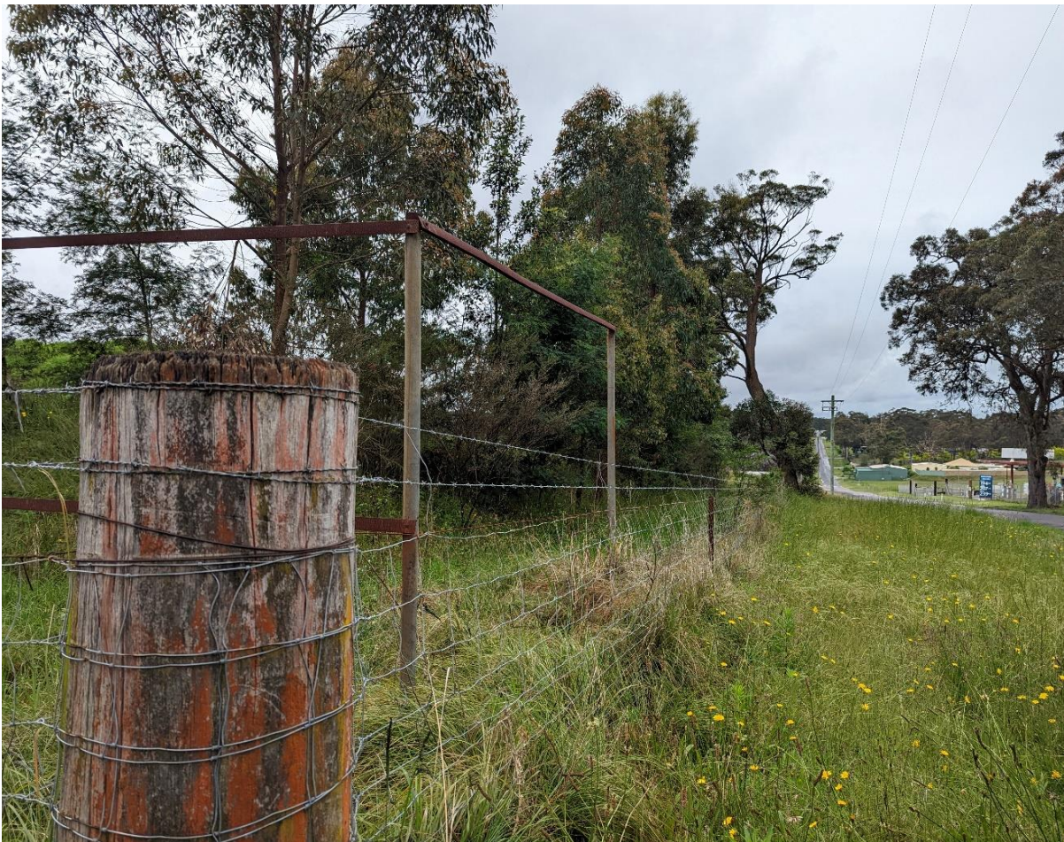
Figure 3. Bund wall adjacent to Roberts Road.
