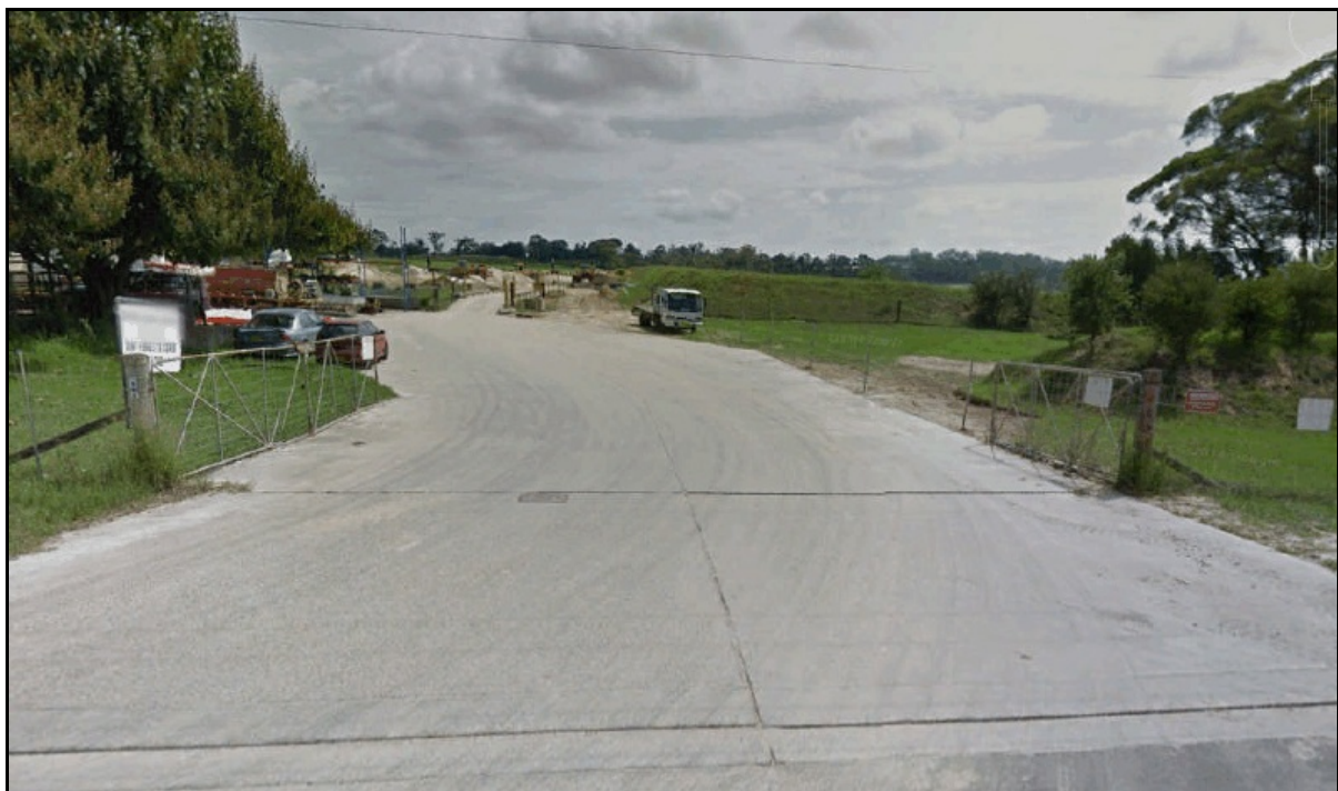
Figure 1.9: This figure shows, at the top view, an aerial photograph of the existing entrance to the Site and the existing weighbridge. At the bottom is a photograph of the existing sealed entrance to the Site with the weighbridge shown in the background of the photograph.
