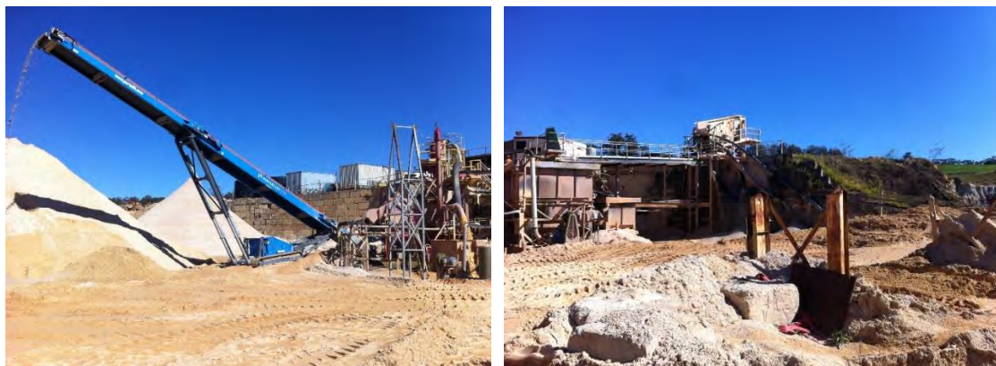
Figure 2-1 Existing Processing Plant
