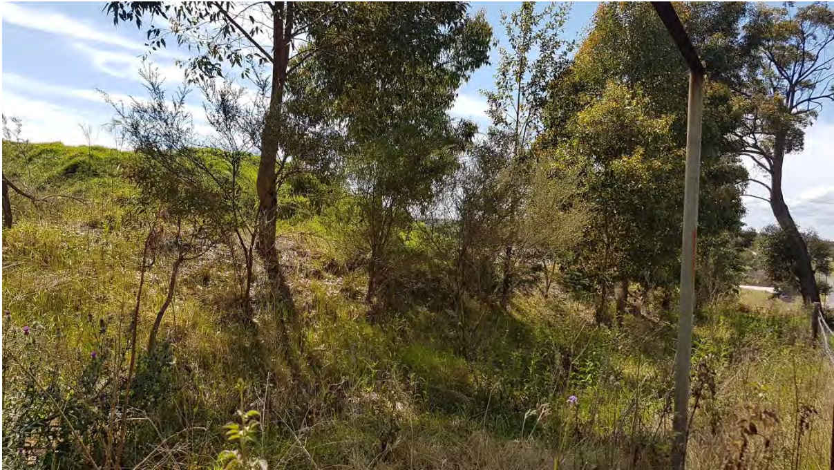
Figure 3. Bund wall adjacent to Roberts Road.
