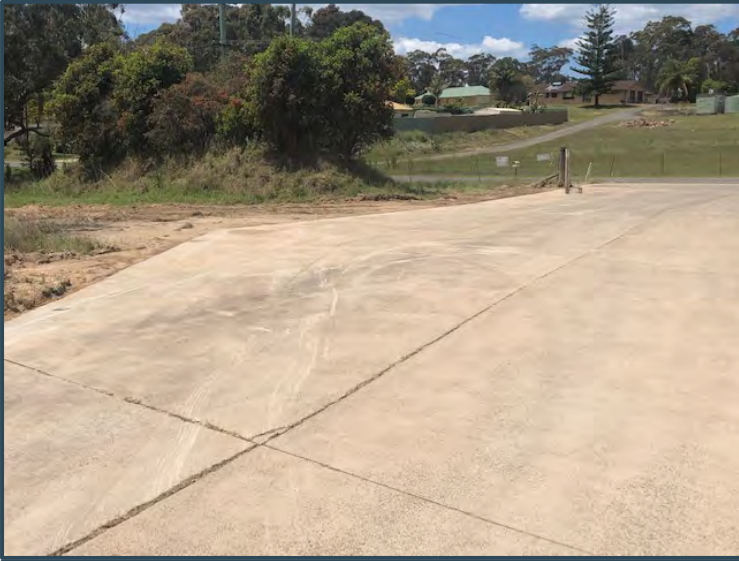
Front gate area 28/10/21
