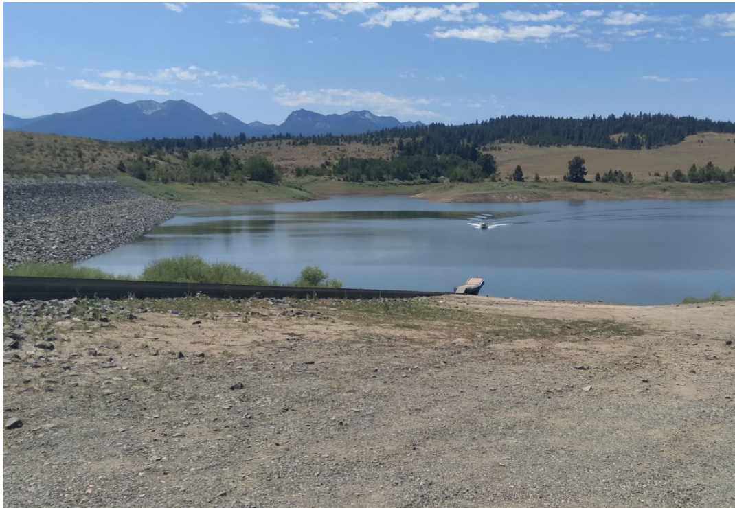
Figure E-13. Wolf Creek Reservoir (Wikipedia, July 6, 2021).
