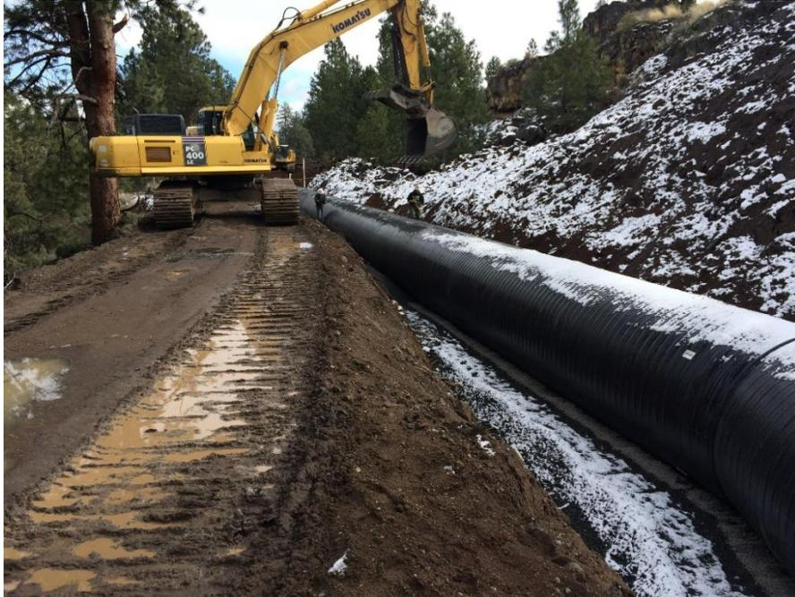
**Figure 6-2. An Example of Construction on a Tumalo Irrigation District Lateral using an Existing Maintenance Road.**
