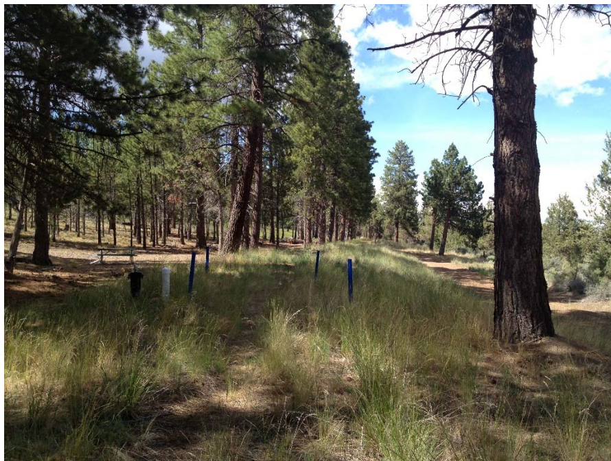
Figure 6-5. A Section of the Tumalo Feed Canal after a Piping Project.
