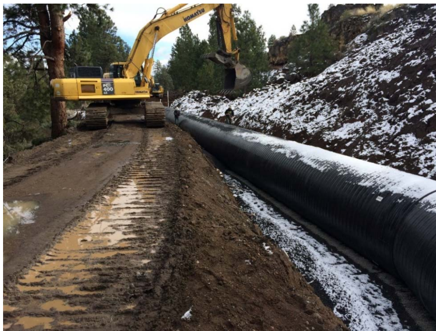
Figure 6-2. An Example of Construction on a Tumalo Irrigation District Lateral using an Existing Maintenance Road.
