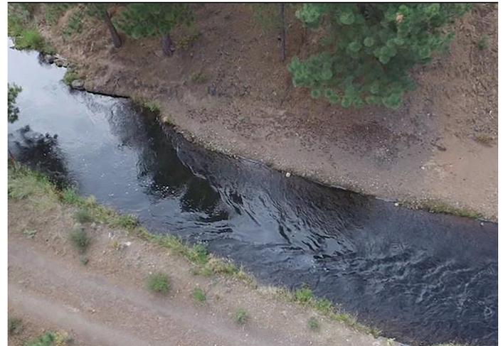
**By converting open irrigation ditches (above) into a closed piped system, Tumalo Irrigation District can reduce water loss from canals by up to 48 cubic feet per second (cfs) or 4.9 billion gallons each season.**
