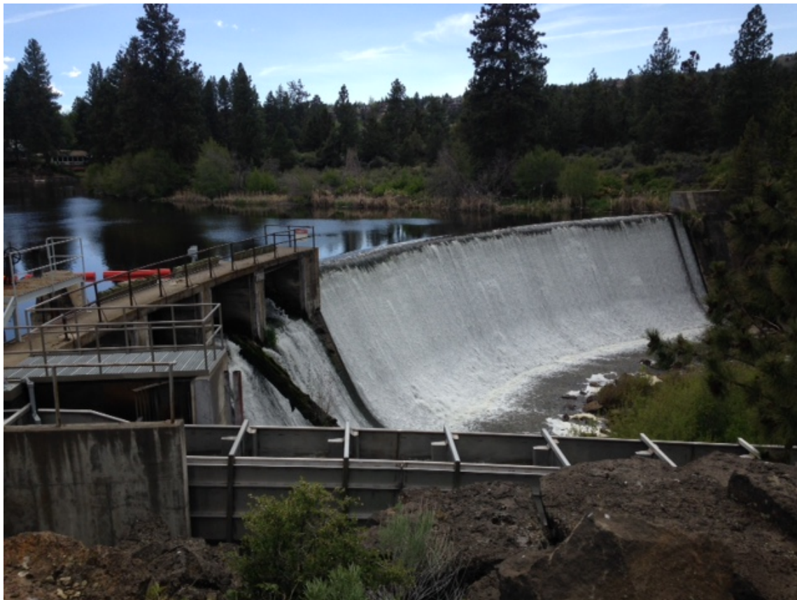
Figure 1-4. North Canal Dam on the Deschutes River (RM 164.8) where Swalley Irrigation District shares an intake structure with Central Oregon and North Unit Irrigation Districts.
