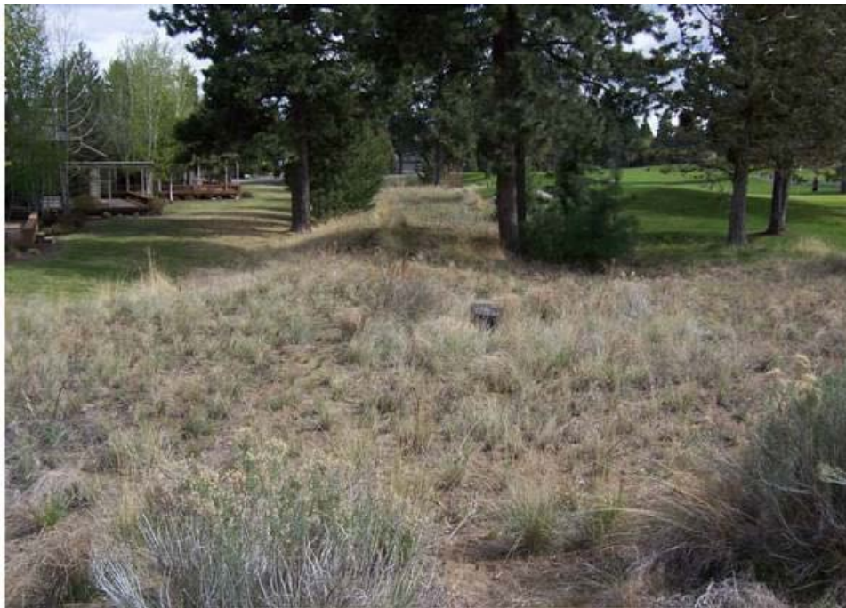
Figure 6-2. A section of the Bend Feed Canal after a piping project.
