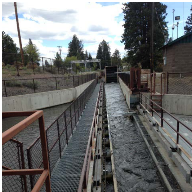
Figure 1-5. The Swalley Irrigation District, Central Oregon Irrigation District, and North Unit Irrigation District fish screen at the North Canal Dam on the Deschutes River (RM 164.8).
