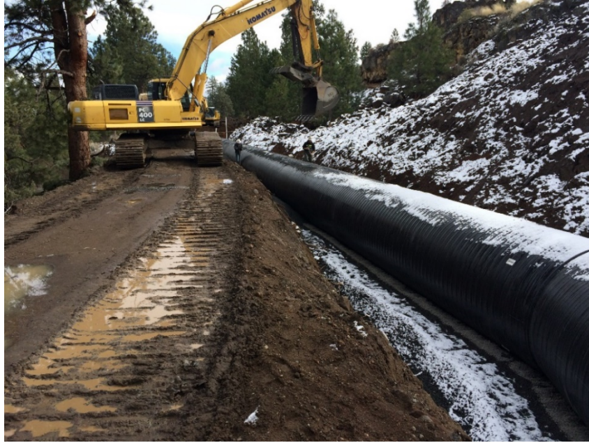
Figure 6-1. An example of construction on a Tumalo Irrigation District lateral using an existing maintenance road.
