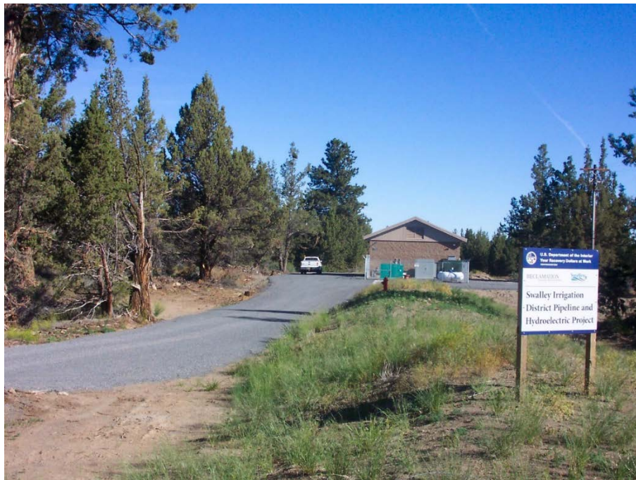
Figure 4-11. Swalley Irrigation District's Ponderosa Power Plant, as seen from U.S. Highway 97.
