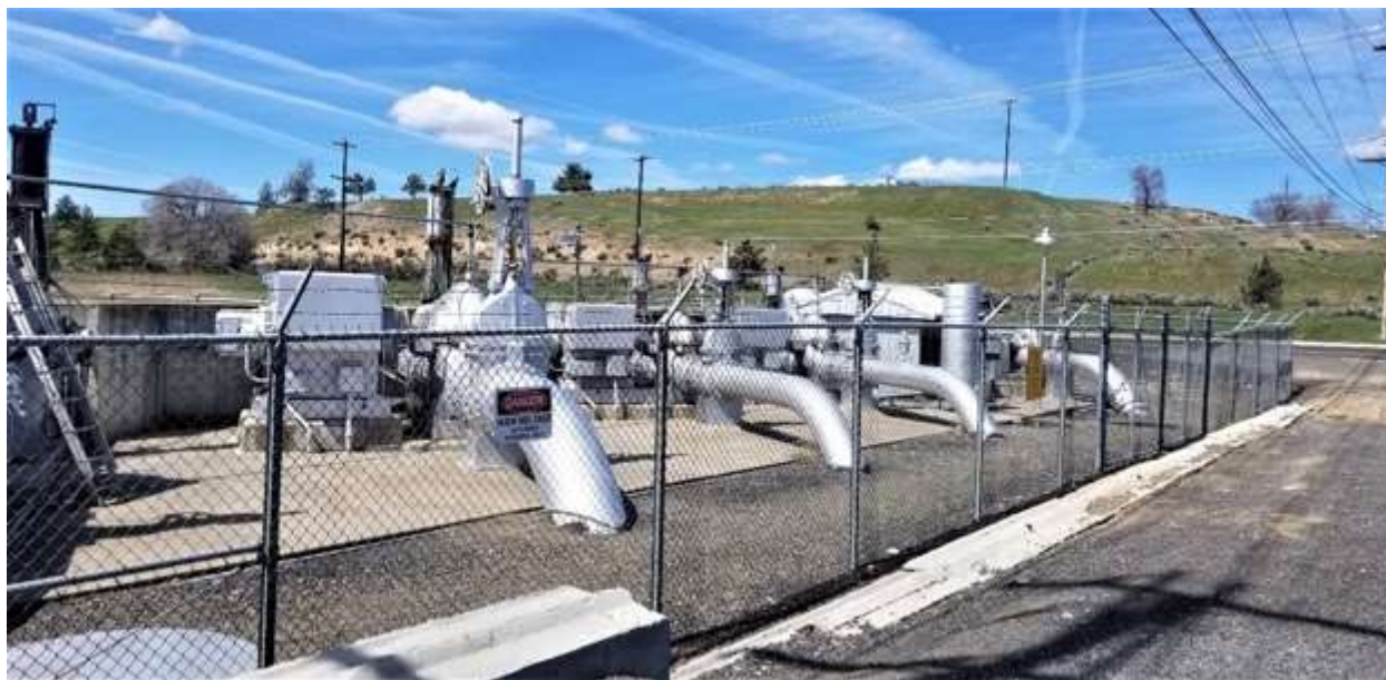
Figure 4-3. The Barnes Butte pump station looking northwest.
