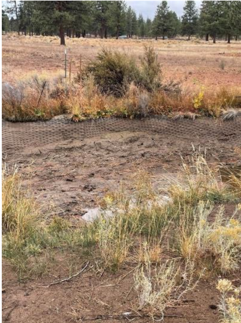
Photograph D-7. Canal lining test section A-7 showing sediment covering the grout-filled mattress, which is difficult and time consuming to remove.
