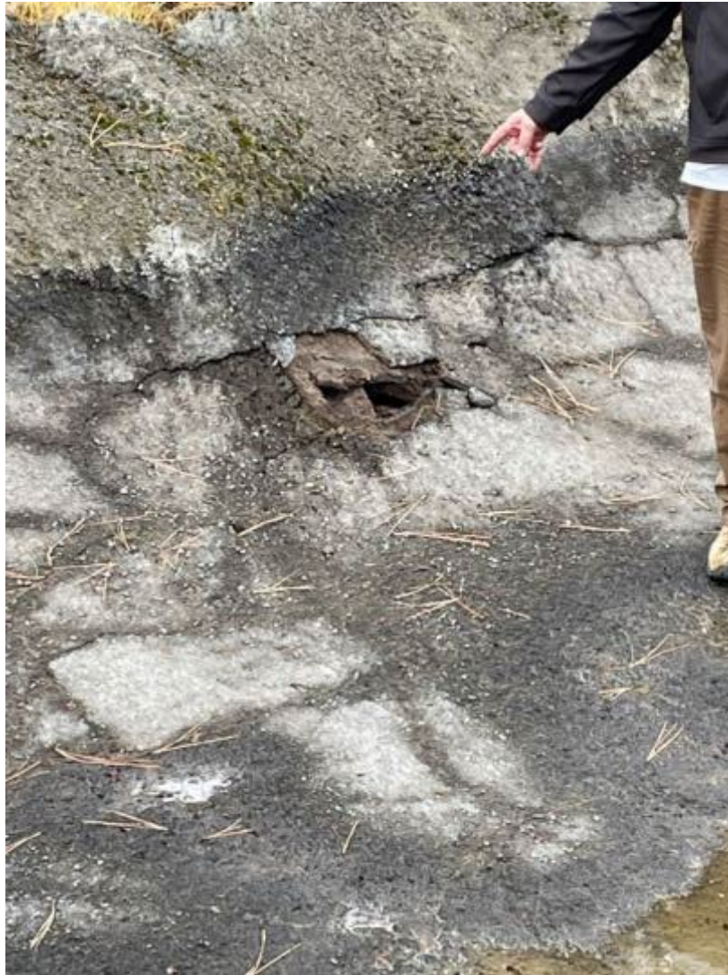
Photograph D-1. Canal lining test section A-1 showing cracks and holes in the shotcrete.
