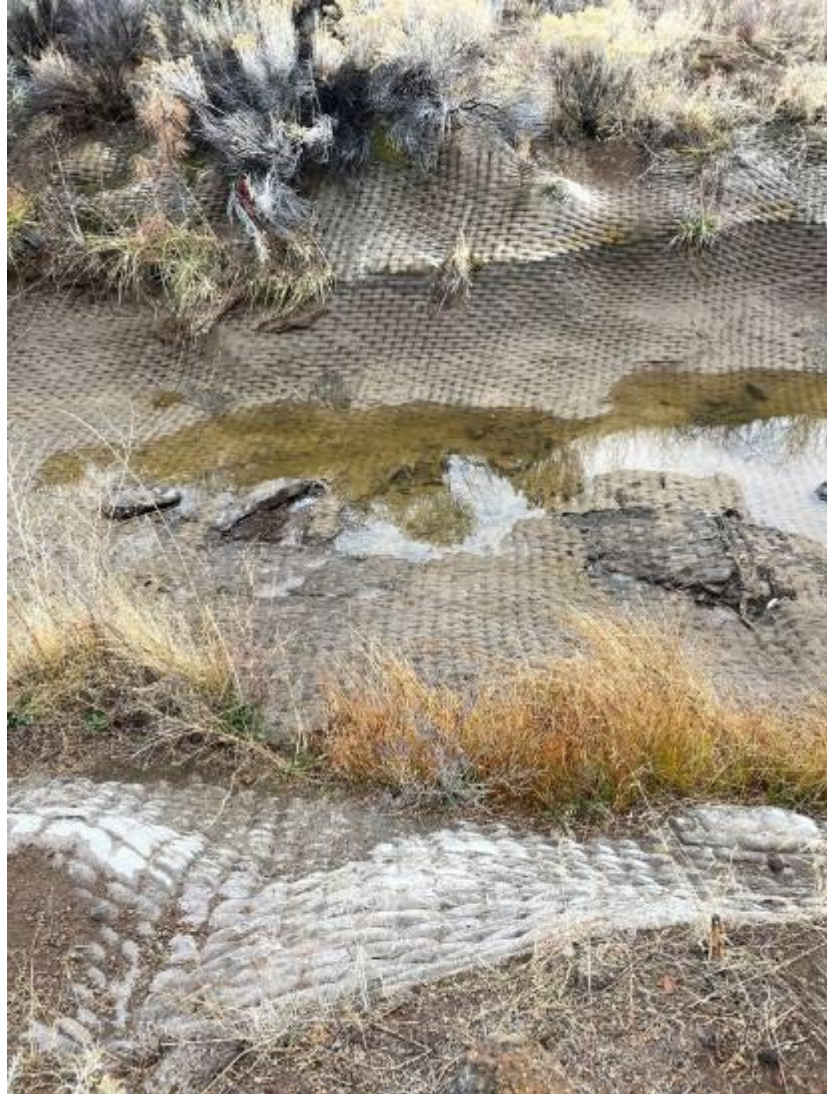
Photograph D-6. Canal lining test section A-7 showing cracking in the grout-filled mattress and vegetation growth.
