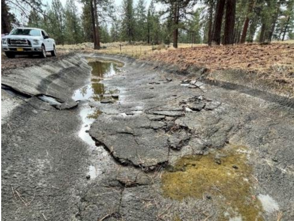
Photograph D-2. Canal lining test section A-2 showing cracks in the shotcrete and broken pieces of shotcrete.
