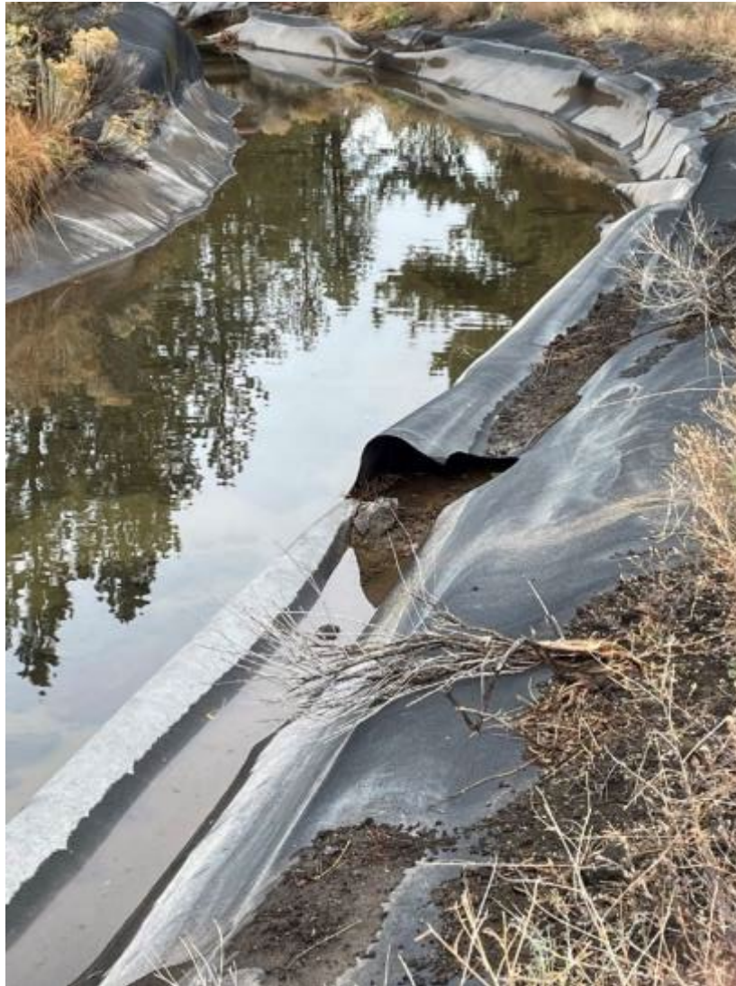
Photograph D-4. Canal lining test section A-3 showing tears in the exposed liner and upwelling of the liner.
