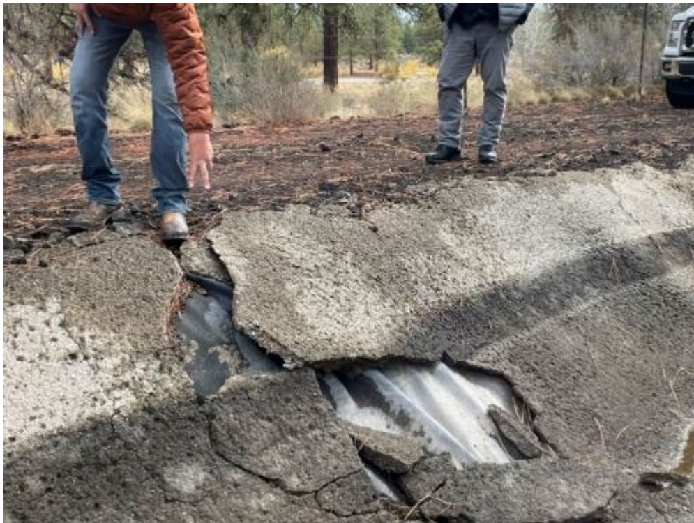
Photograph D-3. Canal lining test section A-2 showing broken shotcrete and exposed liner, which is vulnerable to damage.
