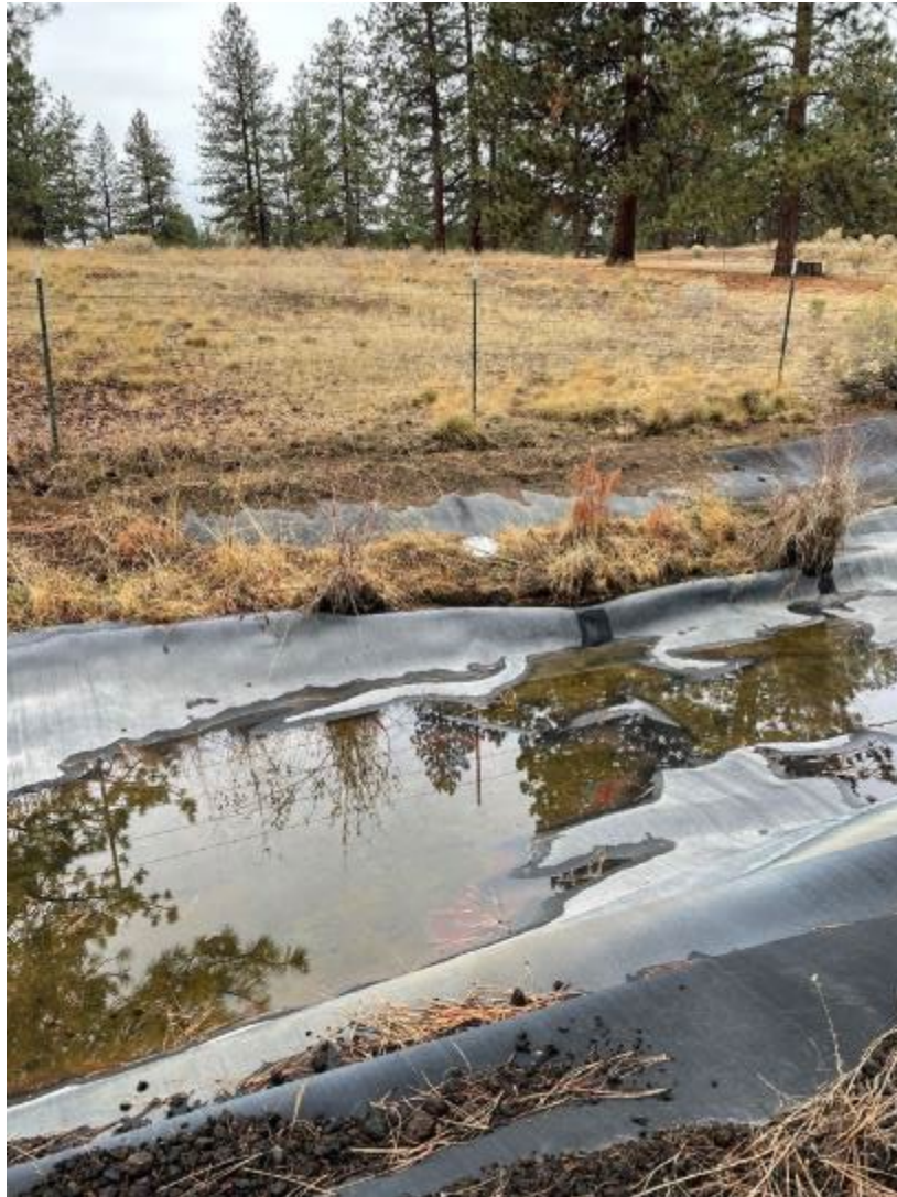
Photograph D-5. Canal lining test section A-3 showing vegetation and debris covering the liner and how the liner has been forced upward, which impedes water flow in the canal.
