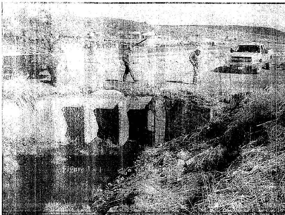
Figure 3 -Typical Triple Box Culvert Crossing
