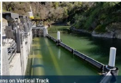
Retrievable T Screens on Vertical Track
