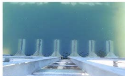
Retrievable Drum Screens on Vertical Track
