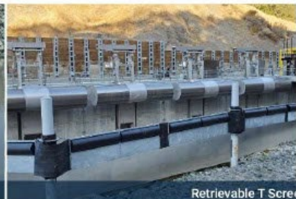
Retrievable T Screens on Vertical Track
