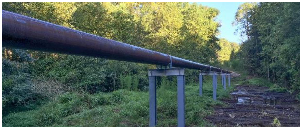
Figure 6-3. A preliminary example of the proposed aerial pipe section of the flume (approximately 450 feet long). The design and materials would be decided closer to implementation.
