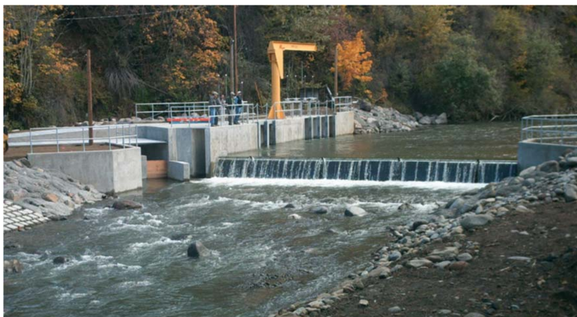
Figure 1-4. The District’s diversion weir, fish ladder, and intake facilities on the East Fork Hood River at river mile 6.6.
