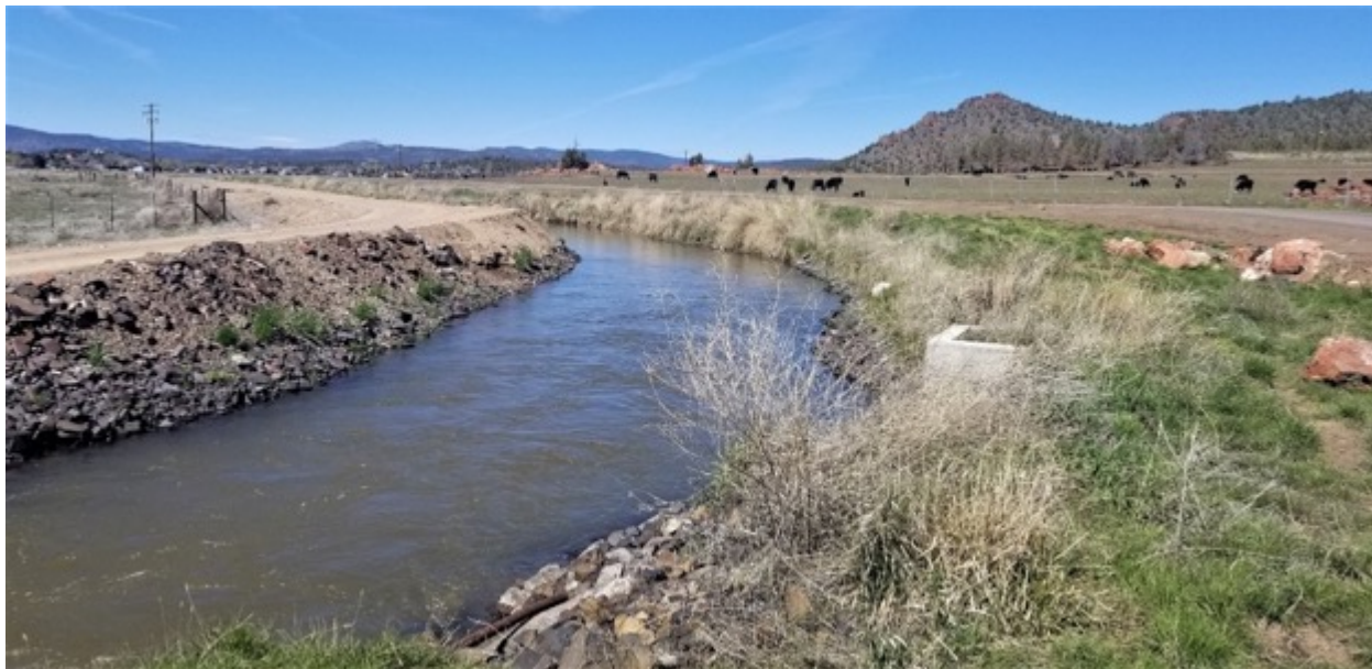
Figure 4-2. IronHorse section of the Crooked River Distribution Canal and canal road looking north.
