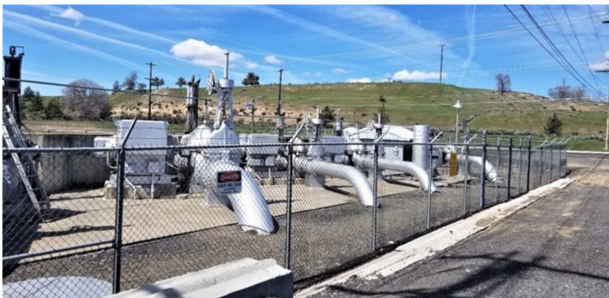
Figure 4-3. The Barnes Butte pump station looking northwest.
