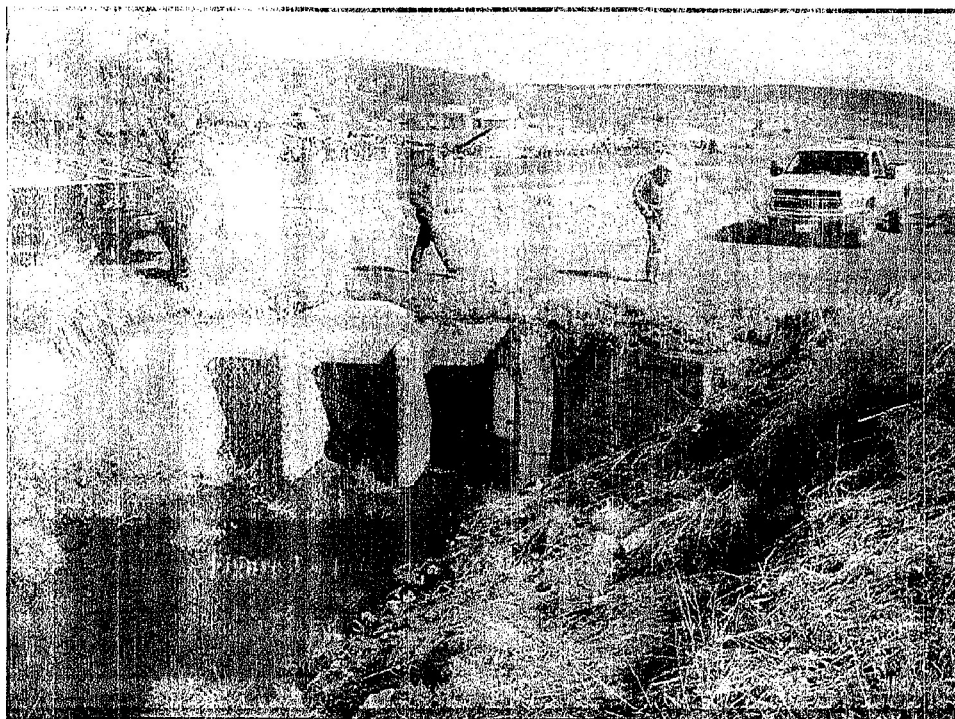
Figure 3 -Typical Triple Box Culvert Crossing
