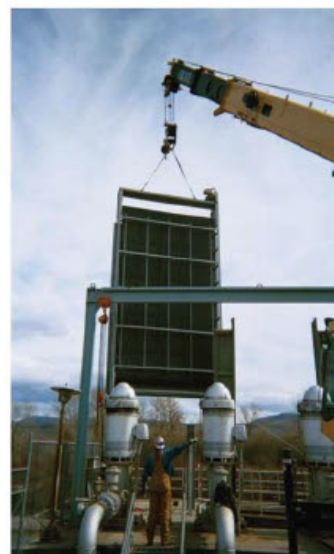
Hydrolox screen as installed at Shell Rock pumping station in the Okanogan Irrigation District.
