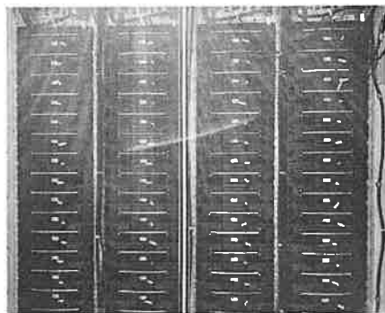
Left: The inside of a container with lithium ion battery stacks. Right: An external view of the battery storage container at a Cypress Creek project in Brunswick, NC. This battery can store 1 MWh of electricity.
