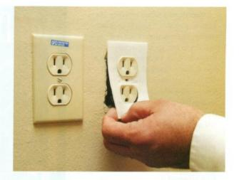
Above: Thomas Marino, president of Advanced Technologies, points out one of the home's smallest energy-saving features: an insulating foam gasket used to prevent air leakage at an outlet plate. The gaskets, which are inexpensive and easy to install, were applied at all switch and outlet plates along exterior walls.
