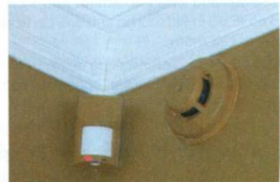
FIGURE 3 One way to blend commercial devices into a home's décor is the careful use of paint. The security provider must oversee this since an uninformed painter may ruin security parts.
