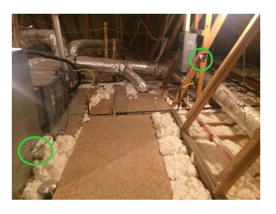
Check for green light. 4 surge protectors to check in upper attic. Both air handlers and 2 water heaters.
