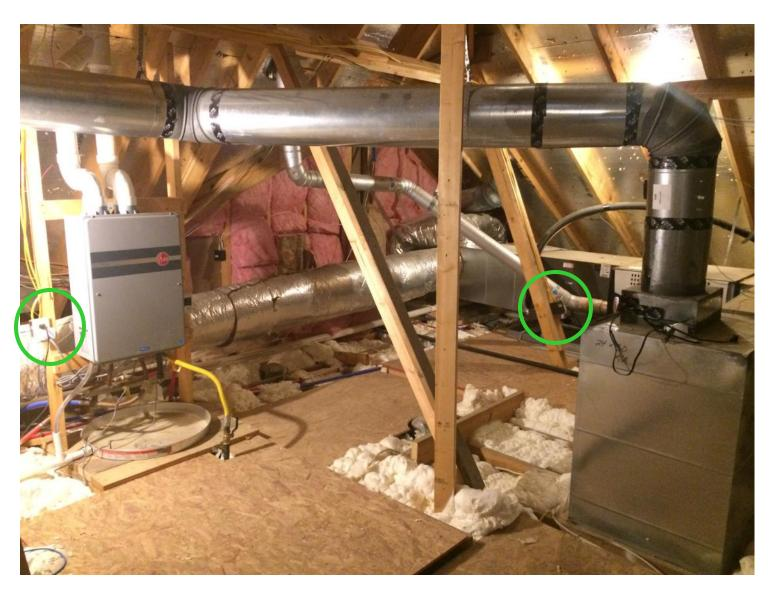
Check for green light. 2 surge protectors to check in Garage attic. 1 air handler and 1 water heater.
