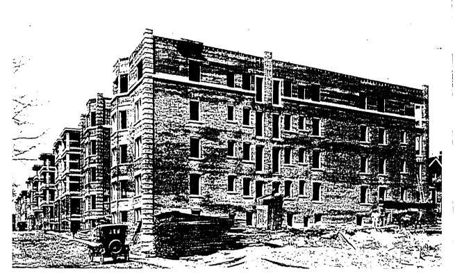
Figure 5: "2,000,000 Bricks in This Pile" — A Row of Eight Apartment Blocks in Various Stages of Construction, Erected by John W. Walker in Kendal Avenue, Toronto [from Contract Record 36 (17 May 1922): 437].
