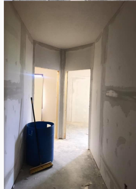
Progress on the Women's Home
