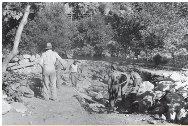
CCC crewmen excavating the site of a spring, July 1935
