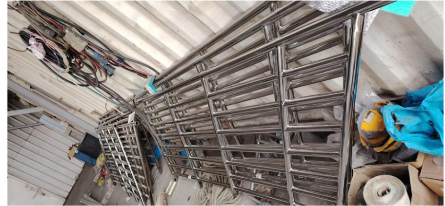
Stainless Steel SS304 Handrail Works
