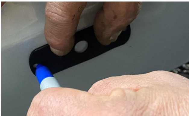
Use the gasket as a template.
